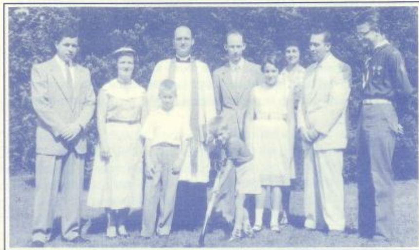
Ground breaking for Fellowship Hall, 1956
